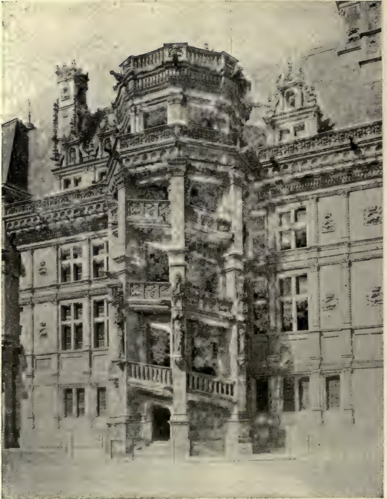
WING OF FRANCIS I WITH STAIRCASE Chateau, Blois
